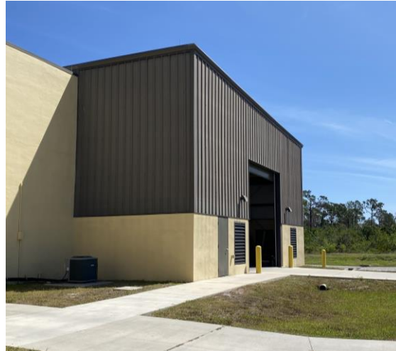
Photo 4-3: RO Expansion Building
